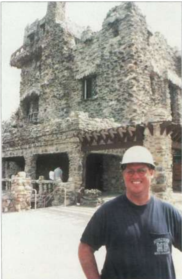
Project supervisor Jim Sabith stands in front of Gillette Castle during the restoration, which took three years and cost $11.5 million. The west and south elevations required repointing, which was "quite an undertaking," according to Sabith, because of the random fieldstone layout. Kronenberger, Sabith's firm, removed and replaced about one inch of the mortar.
