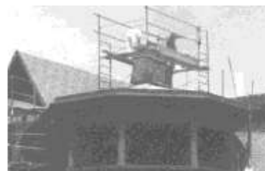
Workers dismantle an existing chimney not original to the House.
