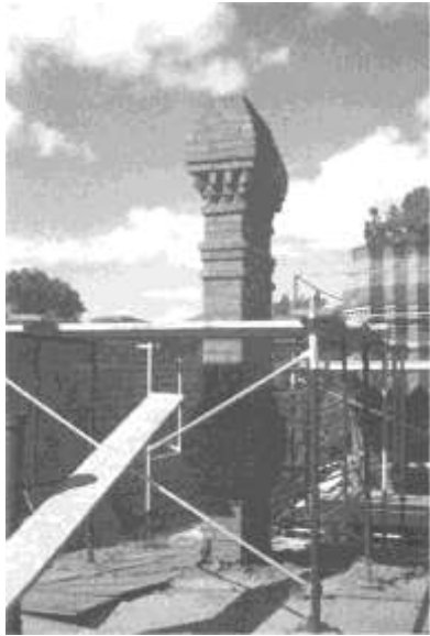
A newly completed fifth chimney rises on the north side of the House. Only four had existed on the House for decades. The design was replicated through digital enhancement of period images.
