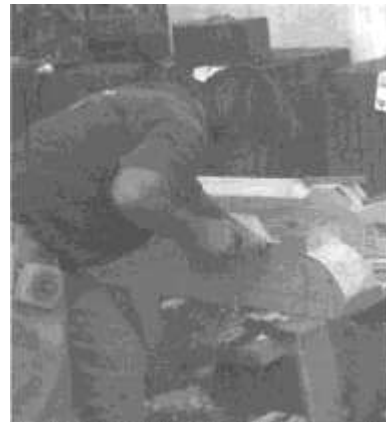
Master carpenter Ihor Budzinski of Kronenberger & Sons creates replacements for damaged wood elements of the House.
