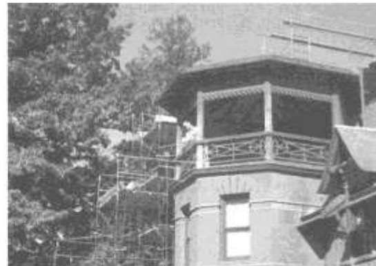
One of the House's several decks is prepared for painting.
