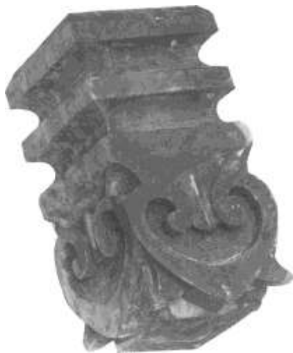
A decorative wood element from the porch of the Billiard Room that was removed for restoration
