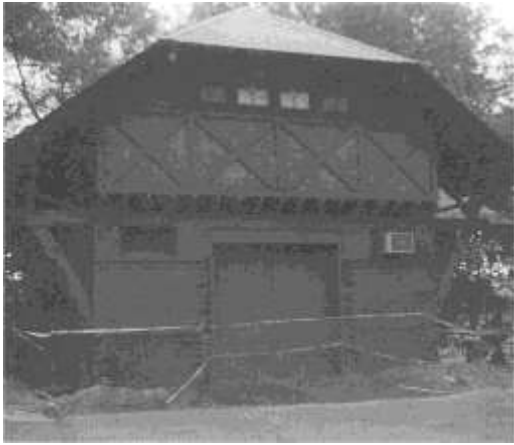
Mark Twain's carriage house before restoration featured wood doors that were installed on the facade in the early twentieth century to accommodate an automobile. The change was made by the Bissell family, who purchased the house from Samuel and Olivia Clemens.
